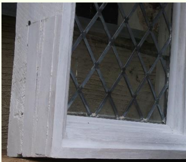
The bottom rail showing the scarf joint on the jamb
