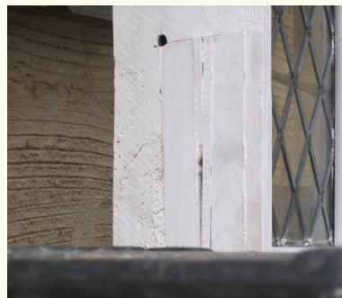
The bottom rail showing the scarf joint on the jamb
