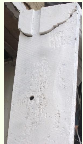
Header joint with jamb
