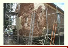
The contractors started removing the old render on Wednesday. The week was extremely hot weather and the task of removing the old render physical and dusty work. While the render crumbled easily where it had delaminated from the cob wall there were places where it was still well adhered. Progress was made on east, south and west elevations during the week. More scaffolding is required to access the wall over the kitchen roof.
