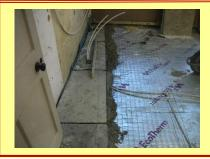
The floor flags are laid on a bed of mortar reinforced by metal mesh. The insulation is laid between the concrete subfloor and the mortar to maximise insulation. The water pipes are laid above the insulation and under the flags.
