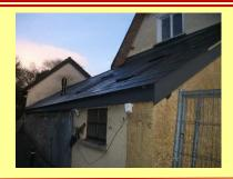
The roof was completed this week with the ridge tiles fitted and all the flashing pointed to make the final seal with the wall. This has enabled the scaffolding to be removed. With the completion of the roof, work has focussed inside.
