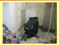
Martin Greenslade, the plumber, has been on site to complete the first fix plumbing. There was a real challenge drilling through the stone wall between the kitchen and store room to enable the pipe work to connect to the boiler.
