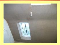
The new plasterboard on the walls and ceiling has been skimmed with a finish coat plaster. The new electrical circuits cables are now hidden with only the tail ends showing on the walls and ceiling. This has enabled work to start on fitting the new flooring.
