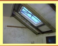
The Velux Roof Windows have been fitted. The windows will enable plenty of natural light to enter the kitchen. The units are double glazed and support our Environmental Policy by reducing heat loss.
