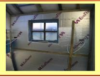
The north facing wall is single skinned of block construction and insulation is now being added located in a timber frame. The insulation will contribute to our Environmental Policy by reducing heat loss.
