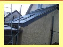
The roof has been covered with a natural recycled slate which supports our Environmental Policy and reflects the local building vernacular. Lead flashing has been used to make a water seal between the tiles and the walls.
