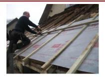
This photograph shows that the old tiles, lathes and felt are stripped from the roof. Mark is working on the roof to fix the new membrane and new lathes.
