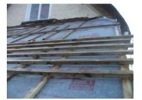
This photograph shows the new membrane has been fixed and the tiling lathes being spaced and fixed.
