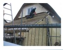
The final lathes are being fixed. Lead flashing will be added to make a water tight seal between the cob wall of the Hall and the new tiled roof.
