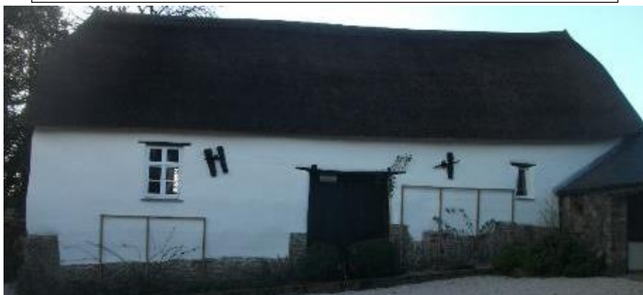
Rear View of Hall Showing Thatch with Overhang
