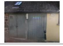
North Elevation. External view showing the external door constructed of single boards with a cross and brace structure internally. Door is poorly fitting leaving many gaps and allowing significant heat loss. Some existing repairs to bottom of door. Other double door is access to self-contained store and not internal to kitchen.
