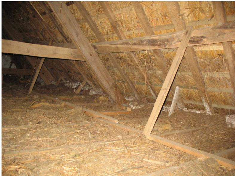
Photograph 6 - Typical truss, purlin and rafter arrangement
