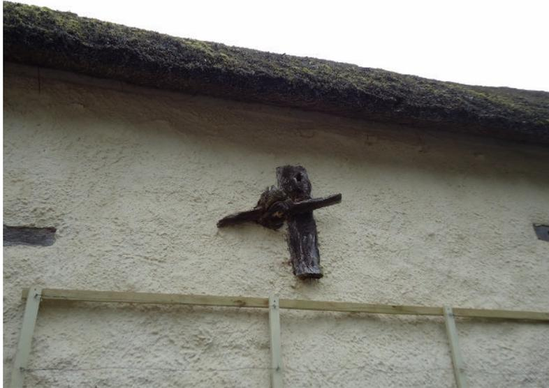
Photograph 5 - Timber tie beams
