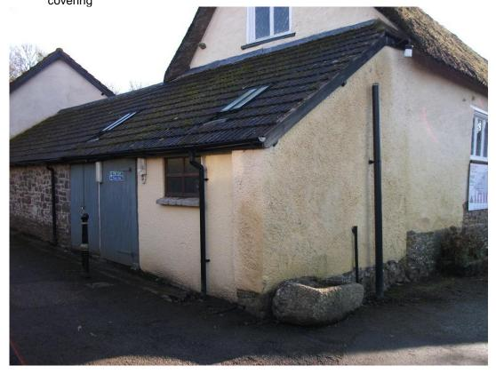
**3.** Side Elevation – (North) – Showing concrete roof covering to be replaced with slate roof covering
