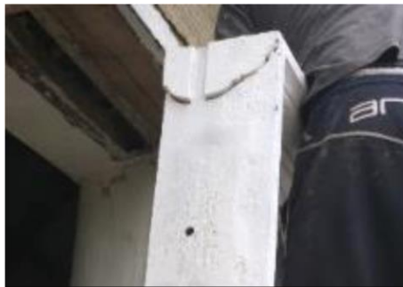
Repairs to the window jamb
