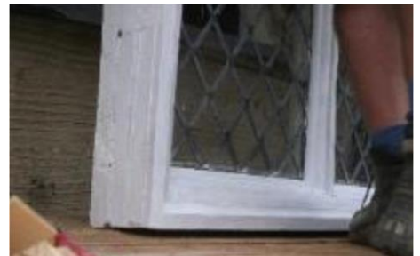
New bottom rail and mullions scarfed into the window
