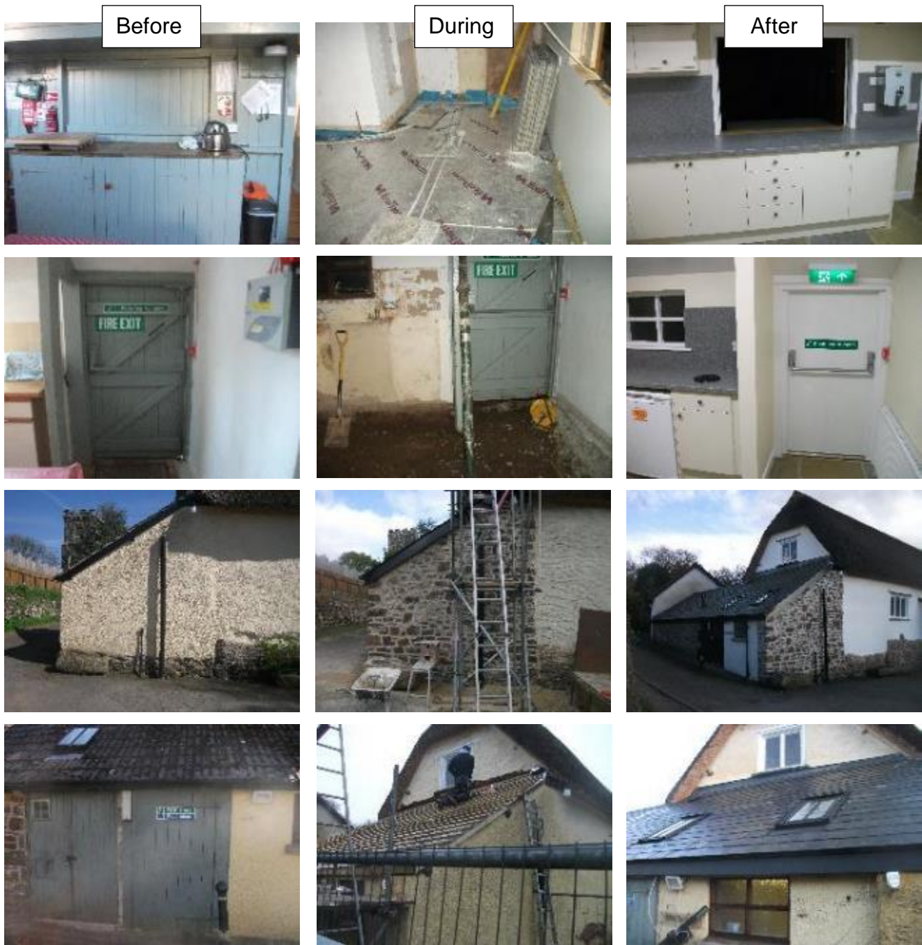
Figure 8 Kitchen Construction: Before, During and After
