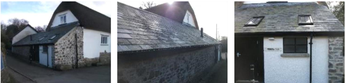
Figure 5 Outside Views of Kitchen from the North Following Conservation Work
