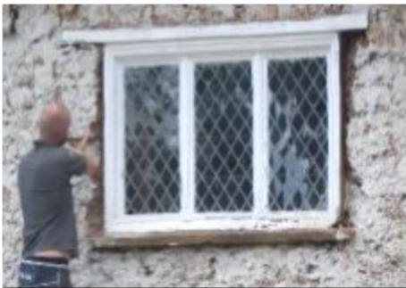
Removing the rotting window
