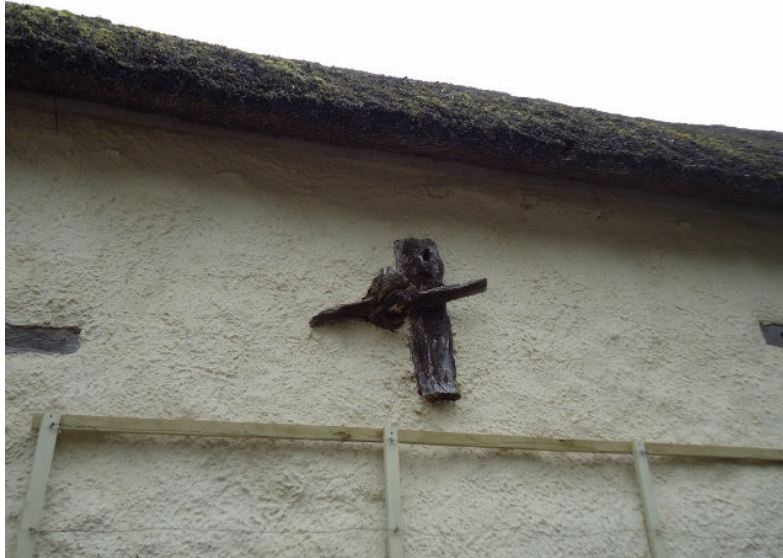
Photograph 5 - Timber tie beams
