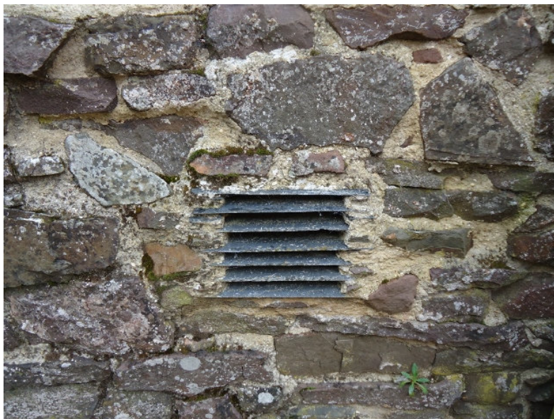
Photograph 8 - Slate vents inserted to aid airflow to undercroft
