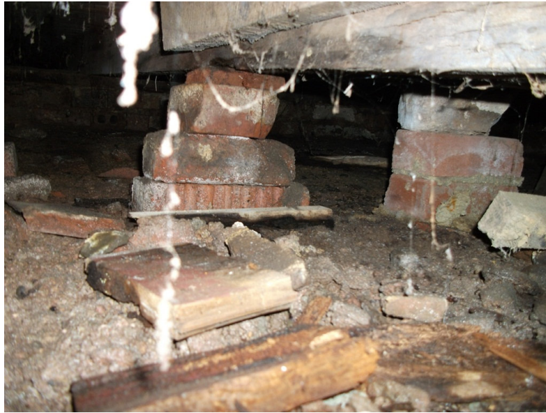
Photograph 7 - Existing undercroft showing raised floor supported on brick piers
