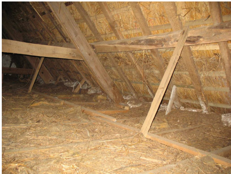
Photograph 6 - Typical truss, purlin and rafter arrangement
