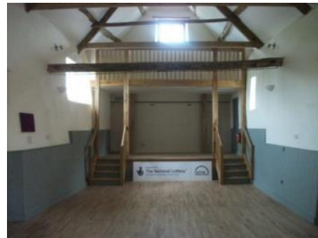
North-facing showing roof construction and exposed window previous hidden
