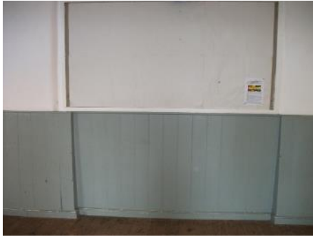
C20th internal partition wall concealing existing old barn door
